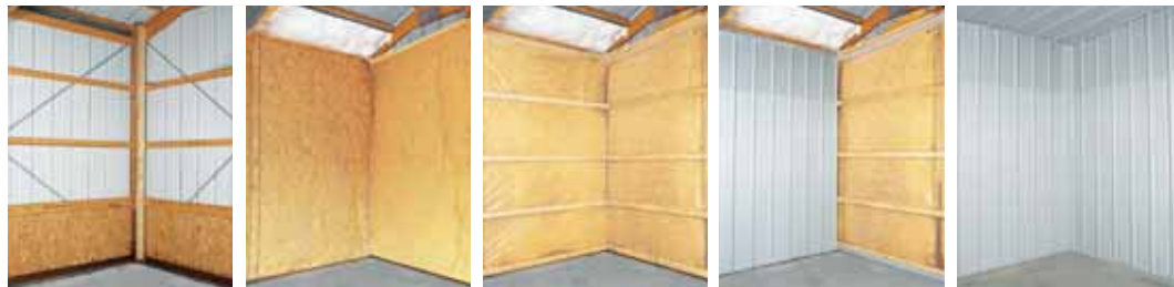
View of corner section before insulation
