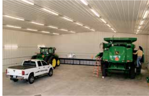
Insulated Machine Storage
